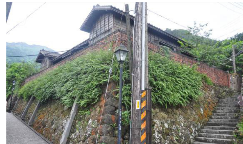
【Image 17】Cement-made facilities showing how mismatched the overall appearance seemed due to the use of cement with the original stones. (Photo captured on June 30, 2014 by Sheng-fa Hsu)
