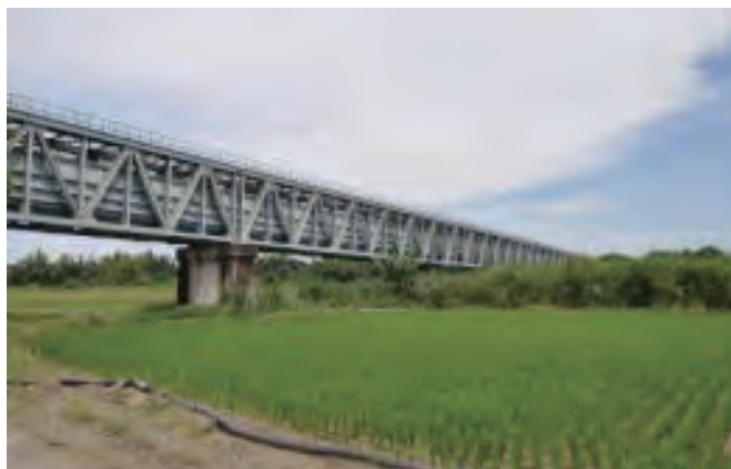
▲嘉南大圳龜重溪渡槽
