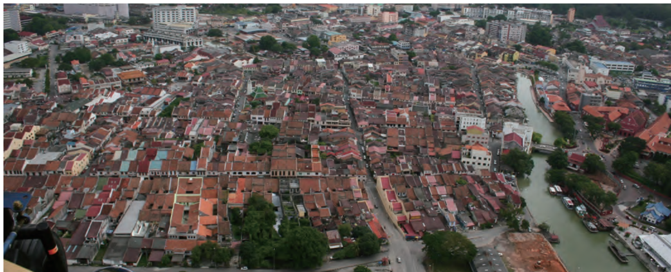
Picture 1 : The overview of Melaka World Heritage Site. On the left is the old residential and commercial area (Asian town) and old administrative area (European town) is on the right separated by the historic Melaka River.
